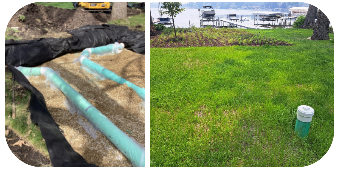
An underground infiltration trench (with observation pipe) during and after construction
