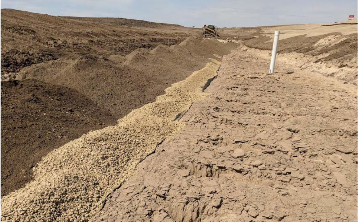
Photo 5: Infiltration basin looking north deep tilled native soil layer with under drain exposed as engineer soil placement commencing
