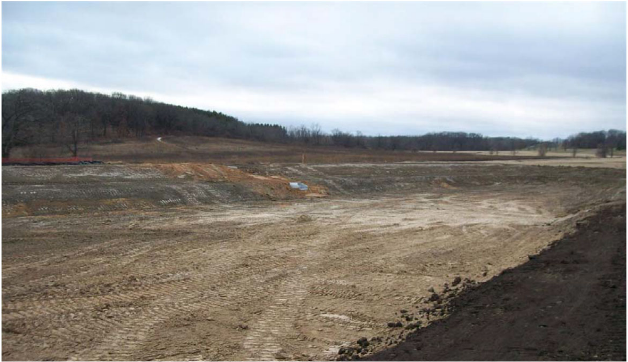
Photo 1: Wet basin looking south west at its initial grading
