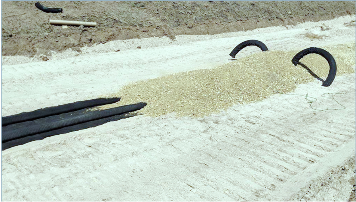
Photo 3: Infiltration basin looking north underdrain configuration
