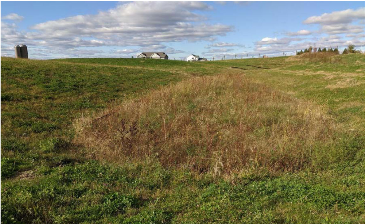
Photo 8: Infiltration basin looking north fully completed after vegetation establishment
