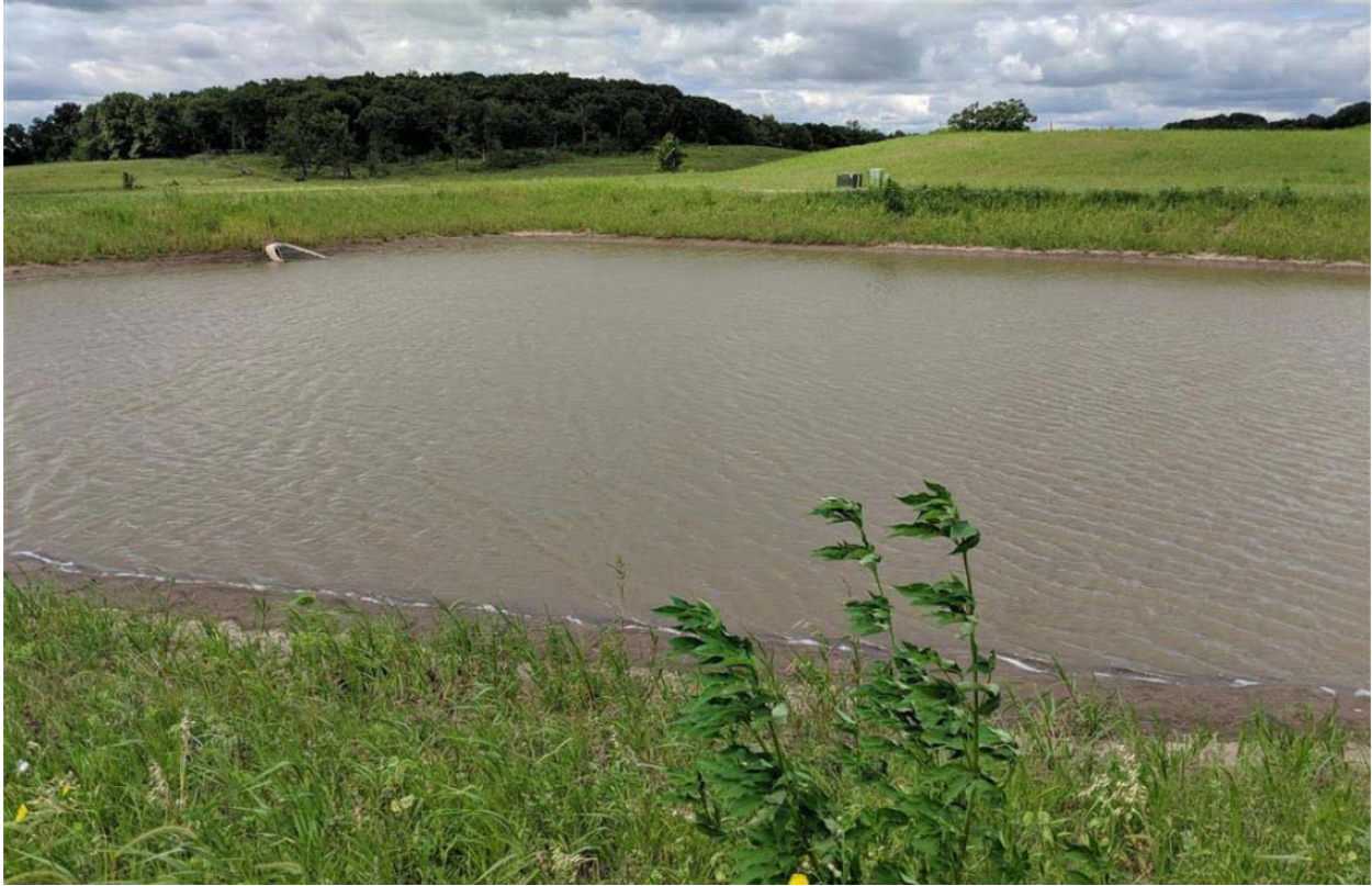
Photo 7: Wet basin looking south west fully vegetated establishment
