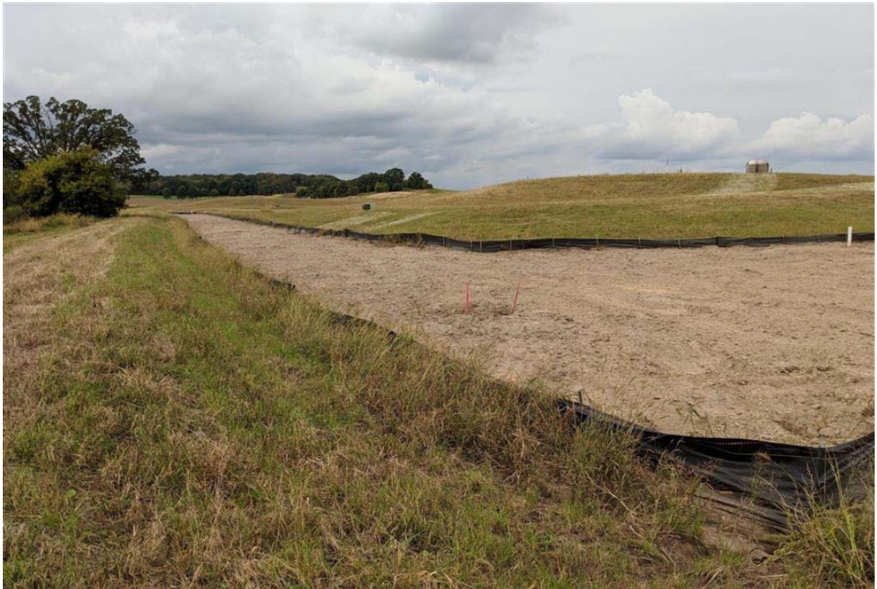
Photo 4: Bioretention basin looking northwest engineered soil prior to final grading and restoration
