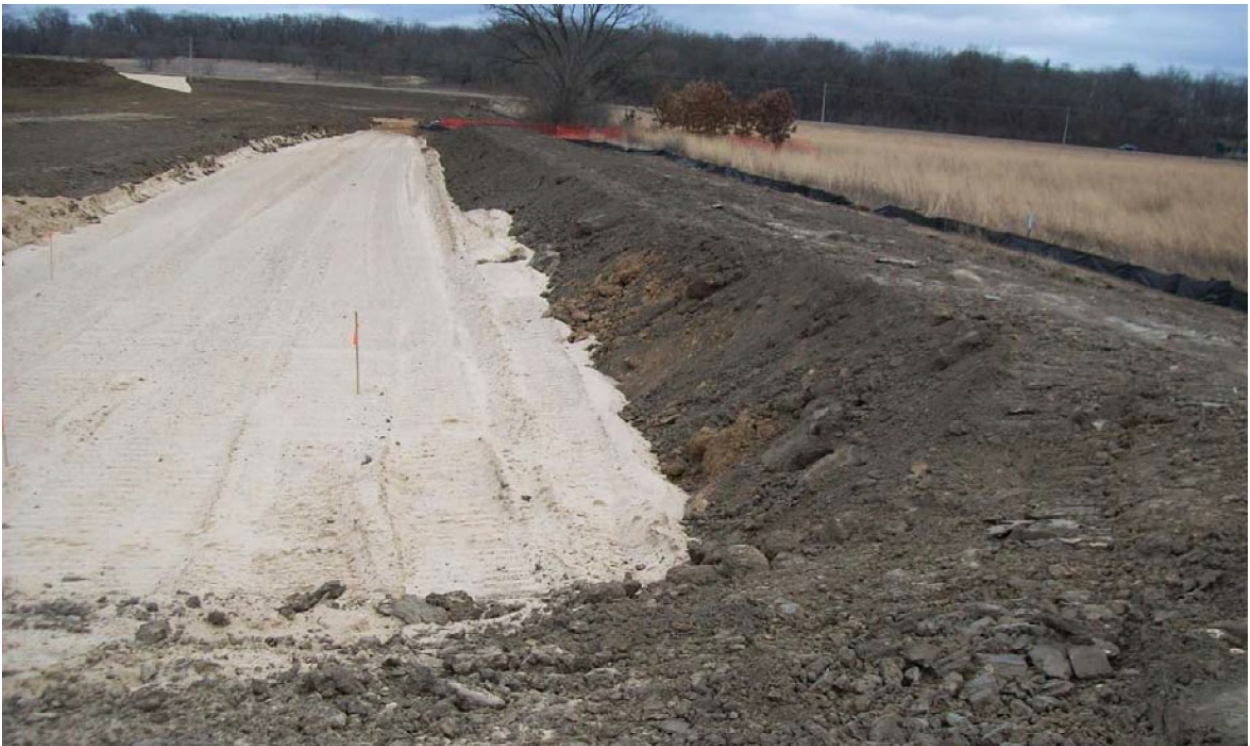
Photo 2: Infiltration basin looking east after undercutting poor soils and replacing with granular soils meeting infiltration requirements.
